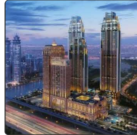
Al Habtoor City, Dubai, UAE Dubai, UAE
