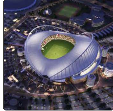
Khalifa International Stadium Doha, Qatar
